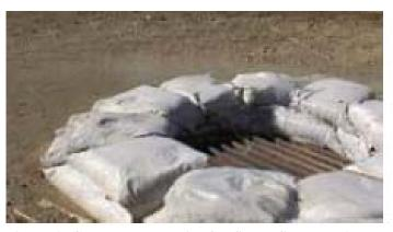
Figure 3 Gravel Bag Barrier for Street Stormdrain Inlets
