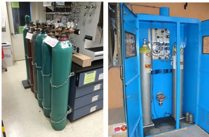
Figure 3.15: Gas Cylinder Storage
