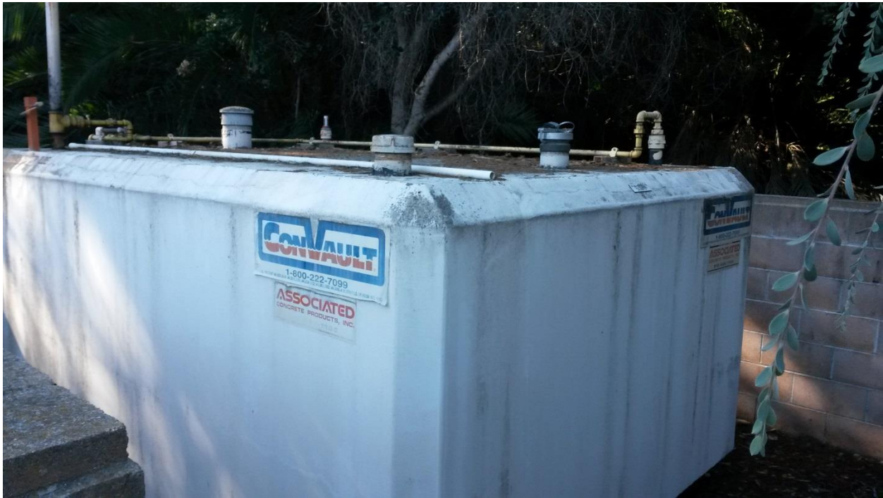
Figure 11- Pump House Diesel Tank, AST-ID 585
