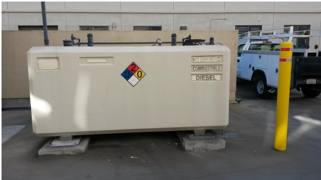
Figure 2- ESB Diesel Tank, AST-ID 225-2
