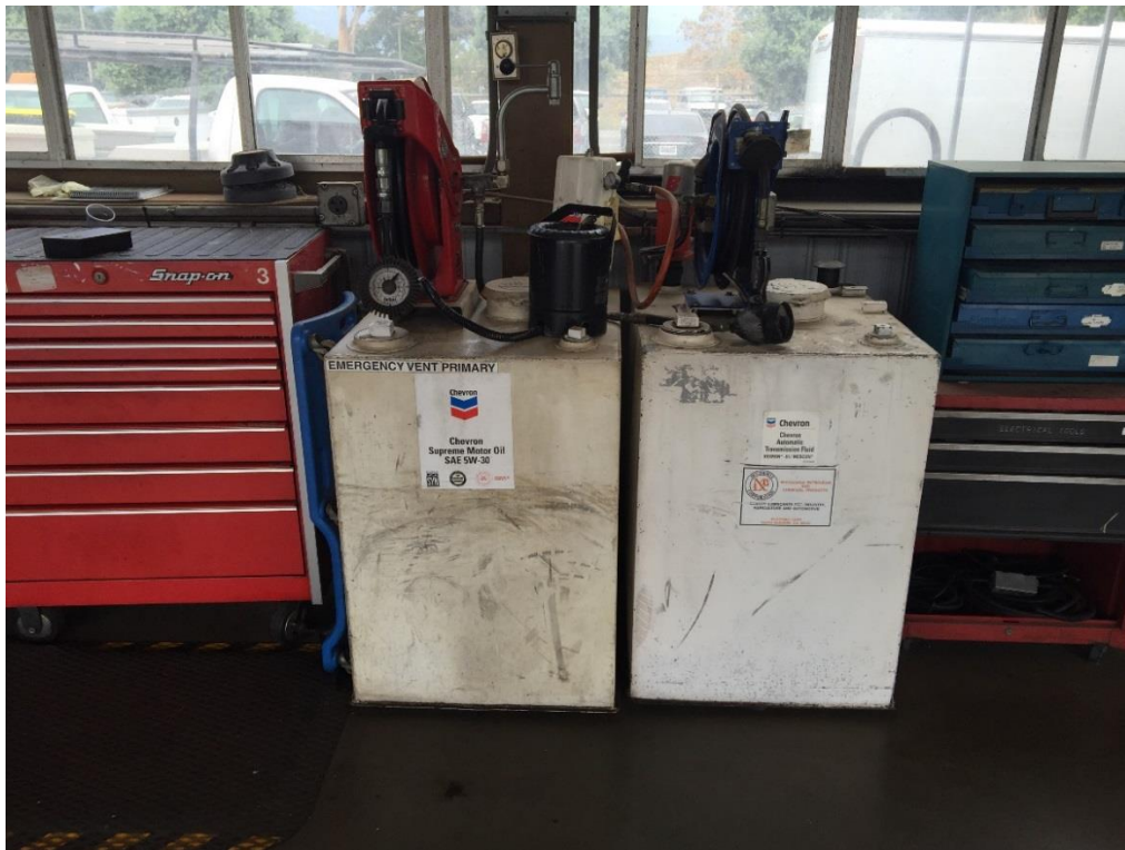
Figure 14- Transportation Services Motor Oil and Transmission Oil Tanks, AST-IDs 595-1, 595-2, 595-6, 595-7
