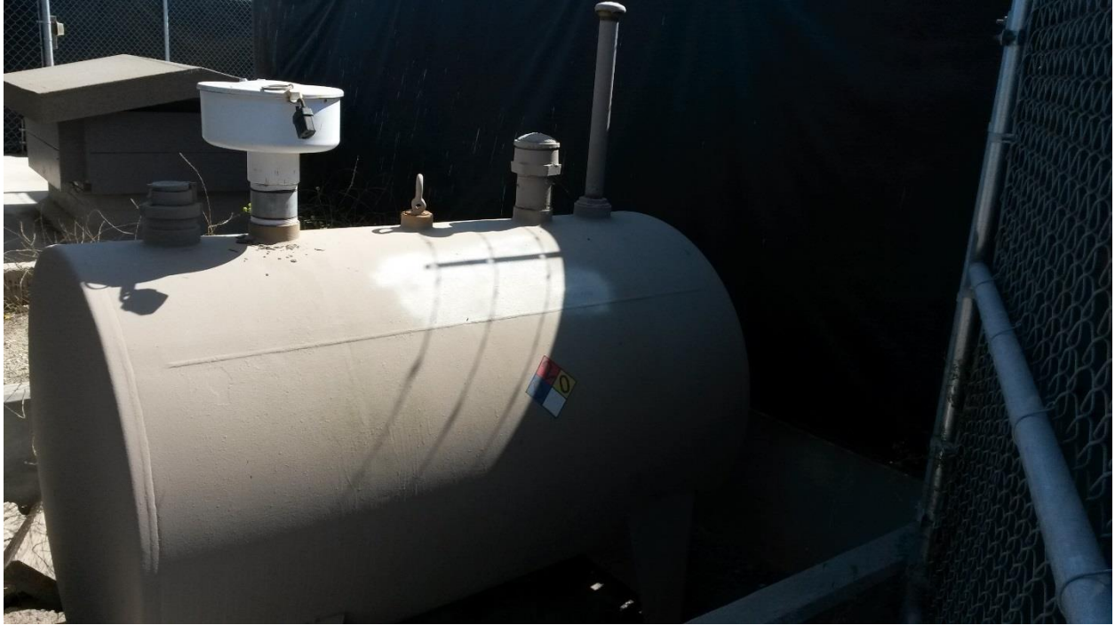
Figure 4- Main Lift Station Emergency Generator Stand Alone Tank, AST-ID 529-2
