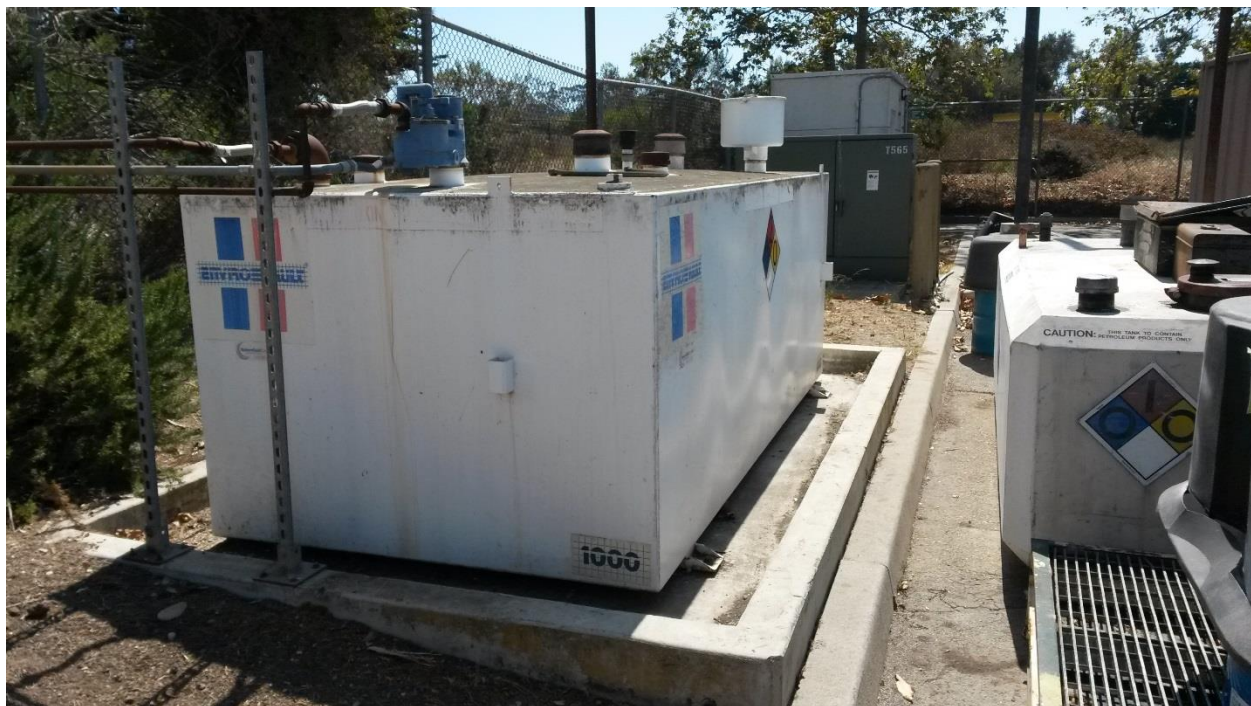
Figure 9- EH&S Emergency Generator Tank, AST-ID 565-12
