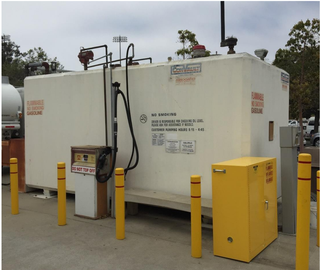
Figure 13- Transportation Services Gasoline Storage Tank, AST-ID 595-4
