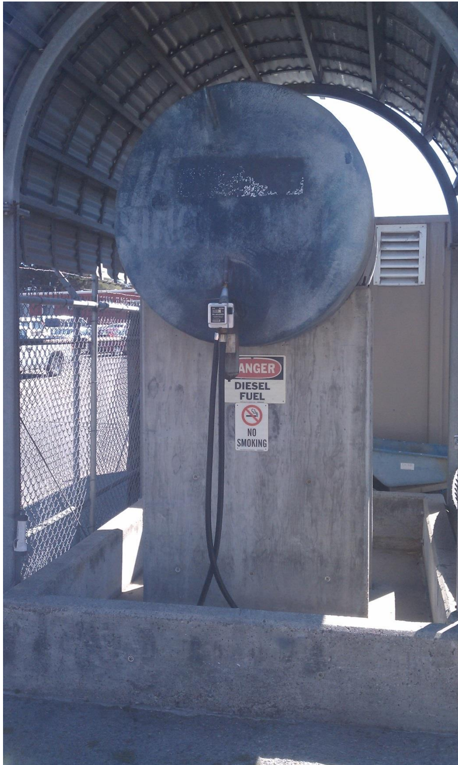
Figure 3- FM Grounds Diesel Tank, AST-ID 340-2
