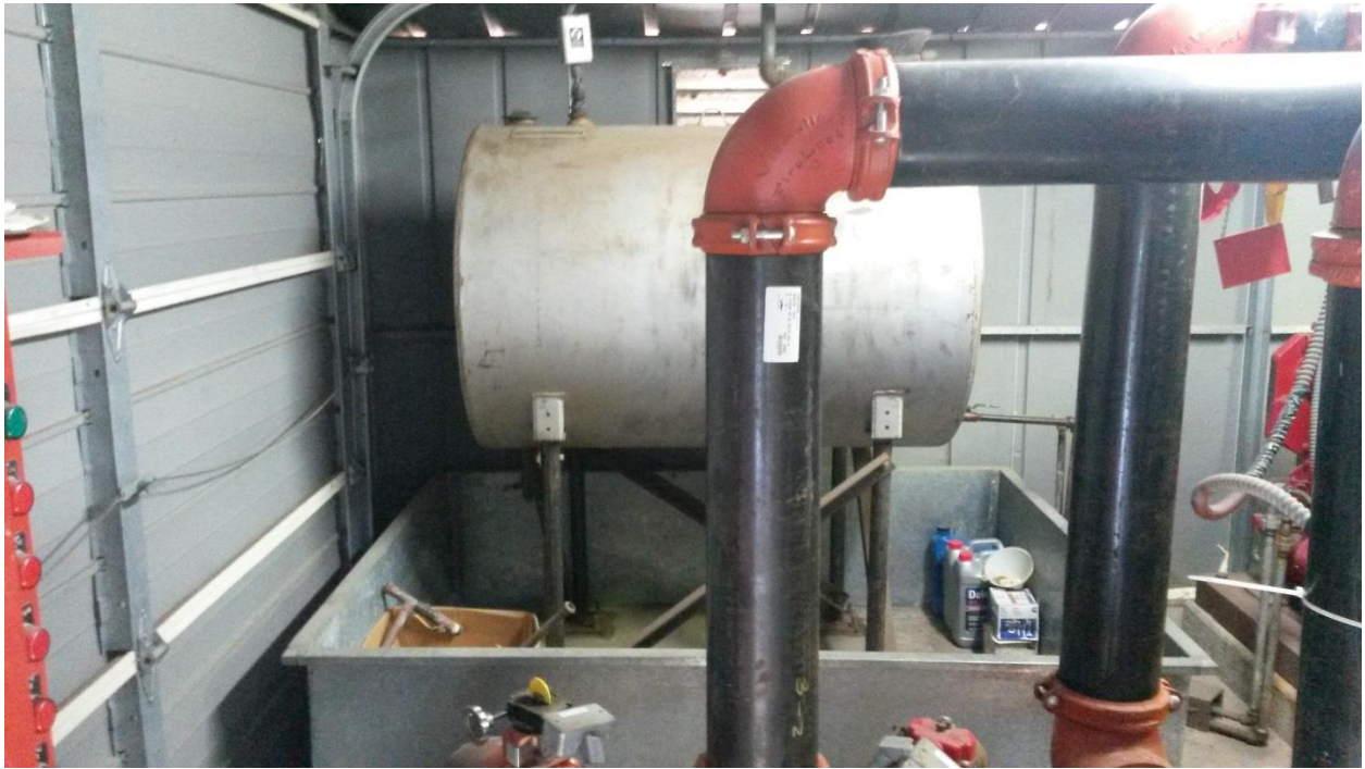
Figure 17– Santa Catalina Fire Pump Tank, AST-ID 860-2
