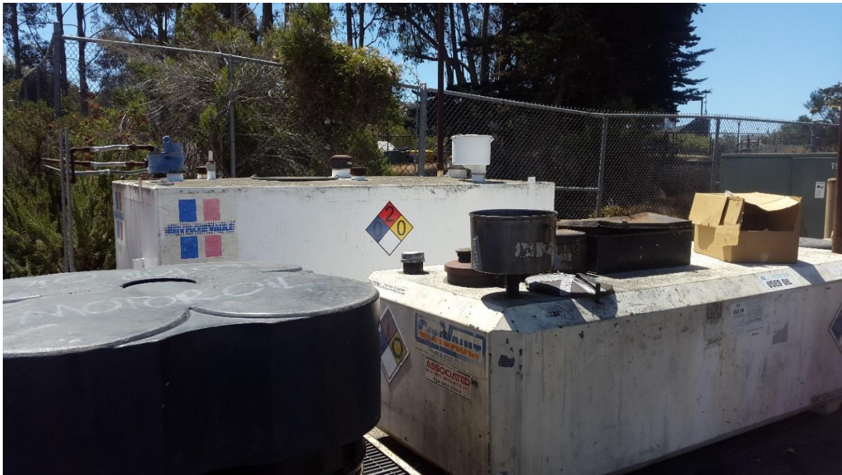
Figure 7- EH&S Emergency Generator Tank (background) and Household Waste Oil Storage Tank (foreground), AST-ID 565-3
