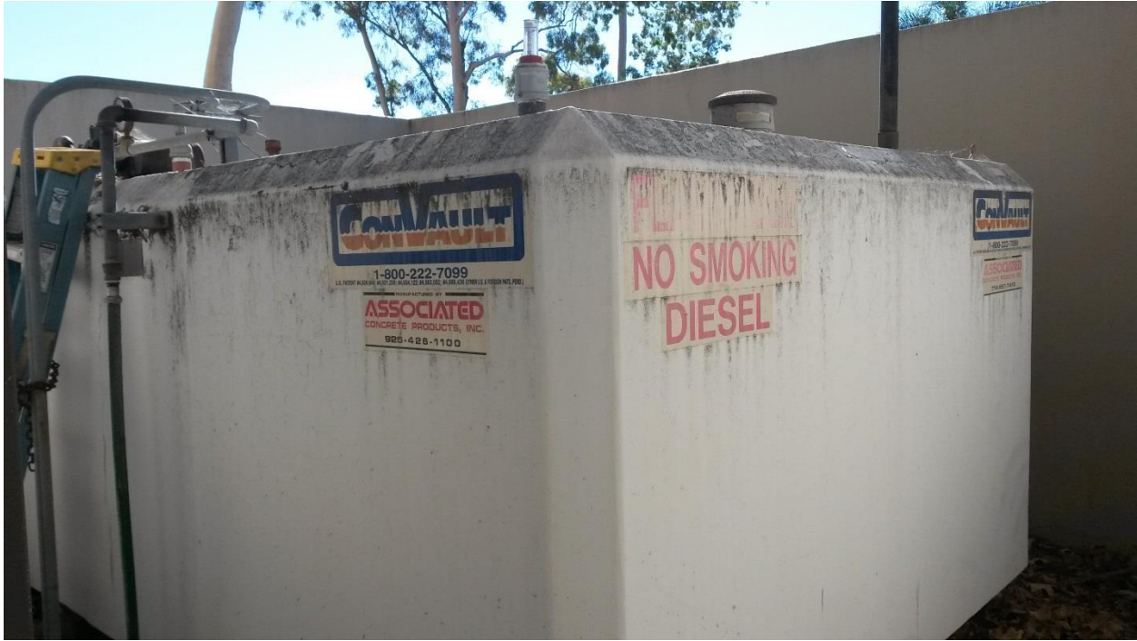
Figure 10- Bio II Diesel Tank, AST-ID 571-2
