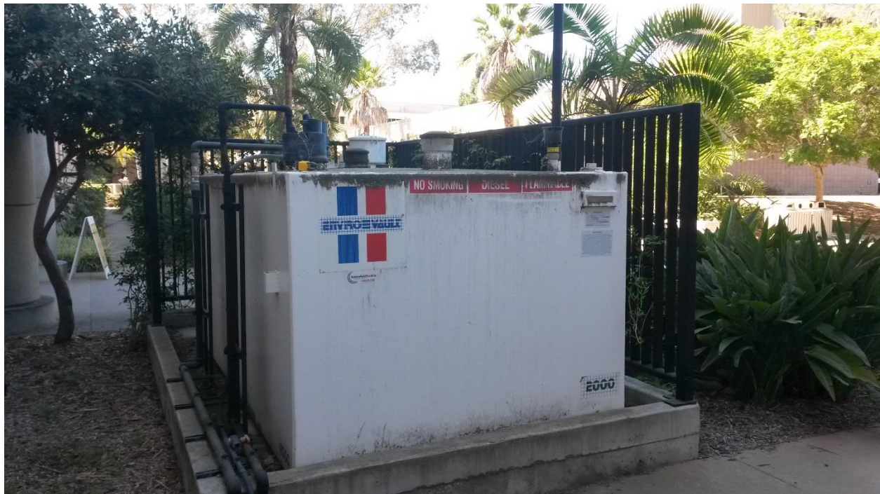
Figure 16- PSBN Emergency Generator Standalone Tank, AST-ID 657-2
