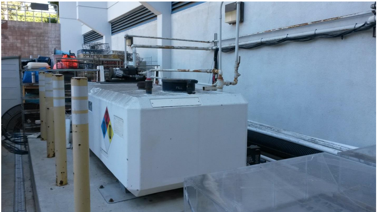
Figure 5- Marine Science Diesel Tank, AST-ID 555-4
