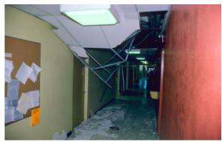
The shock wave from the blast continued up through the hood ductwork and into the corridor where a secondary explosion blew out the false ceiling panels.
