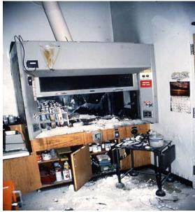
The fume hood was seriously damaged. Note the damage to the hood back wall and how the ductwork above the hood is askew. Note also the gas lecture bottles which could have been compromised - hoods should be for chemical use, not chemical storage.
