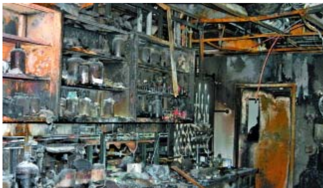
DESTROYED Coleman's lab after the April 8 explosion and fire at Ohio State.
